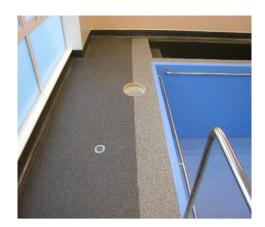
**Decorative Supascreed** made with increasing levels of coloured quartz aggregates. Please note that the cost of the system increases with aggregate concentration.
