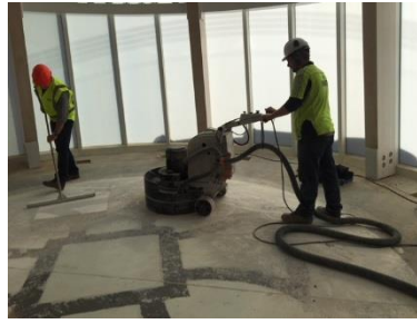
Grinding Process underway
