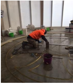
Installation of Brass Strip
