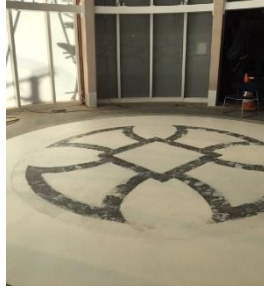
Architectural Terrazzo has been installed
